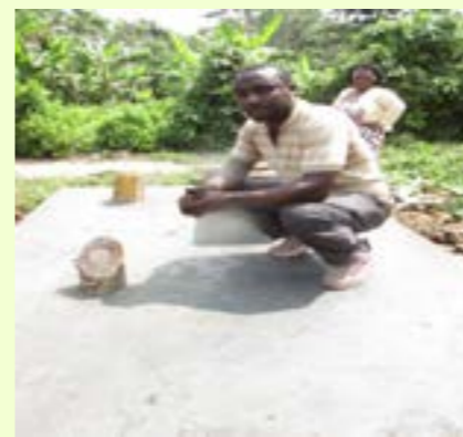
Slab under construction
